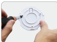
5. Fix the magnetic clasp with screws on the ceiling or the wall.
