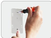
2. Fix the magnetic clasp with screws or sponge rubber on the wall
